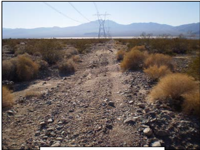
Section 10-View to the west Power line access road
